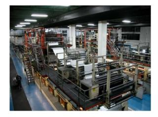
**Solution:** Dynamic V-Banks and Dynamic V8 Air Cleaning Systems. Dynamic V-Bank Air Cleaners were installed in twelve 4' x 4' drop return duct inlets inside the printing bay. Downstream of the V-Banks, Dynamic V8 Air Cleaning Systems were installed in a mixed air
