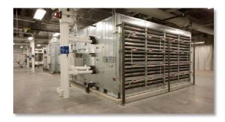
**Solution:** Dynamic V8 Air Cleaning Systems (no pre-filters) were installed in the air handling units (pictured above).
