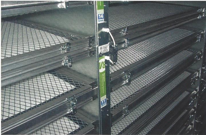
Polarized-media electronic air cleaners.
